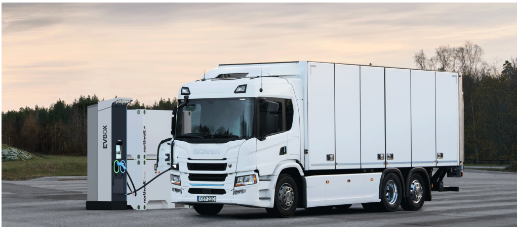
Figure 2.3.: A collaboration between Northvolt, Scania and EVBox, using a BESS in conjunction with heavy electric vehicle charging. [26]
